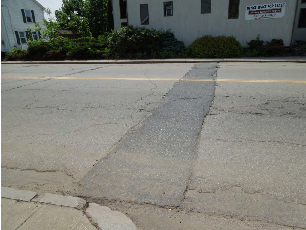
AUBURN STREET – SIDEWALK, GRANITE CURBING, STRIPING AND PAVEMENT CONDITIONS
