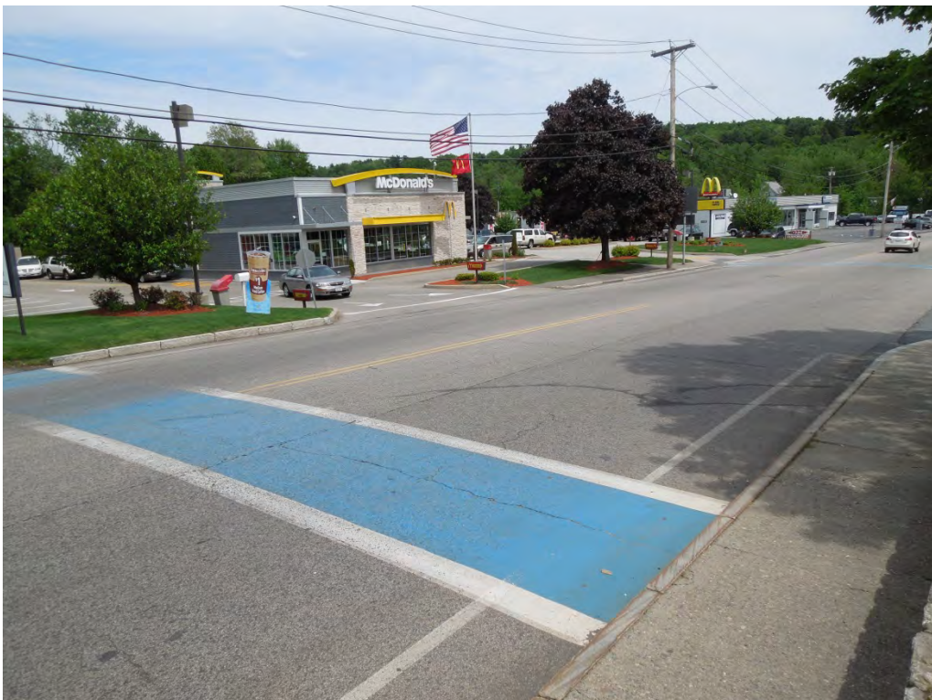
AUBURN STREET – CROSSWALK NORTH OF HIGH SCHOOL ENTRANCE (ADA ACCESSIBILITY ISSUE)
