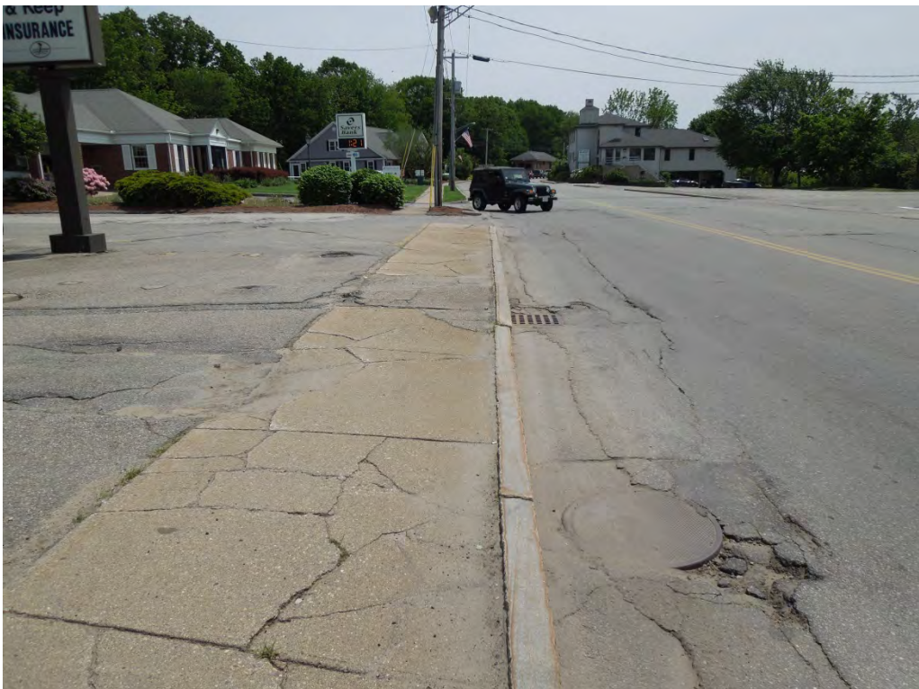
AUBURN STREET – SIDEWALK, GRANITE CURBING, STRIPING, DRAINAGE, PAVEMENT CONDITIONS
