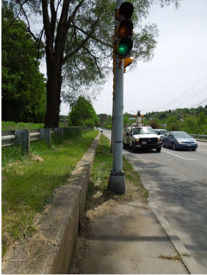
AUBURN STREET TRAFFIC SIGNAL AT BROTHERTON WAY INTERSECTION
