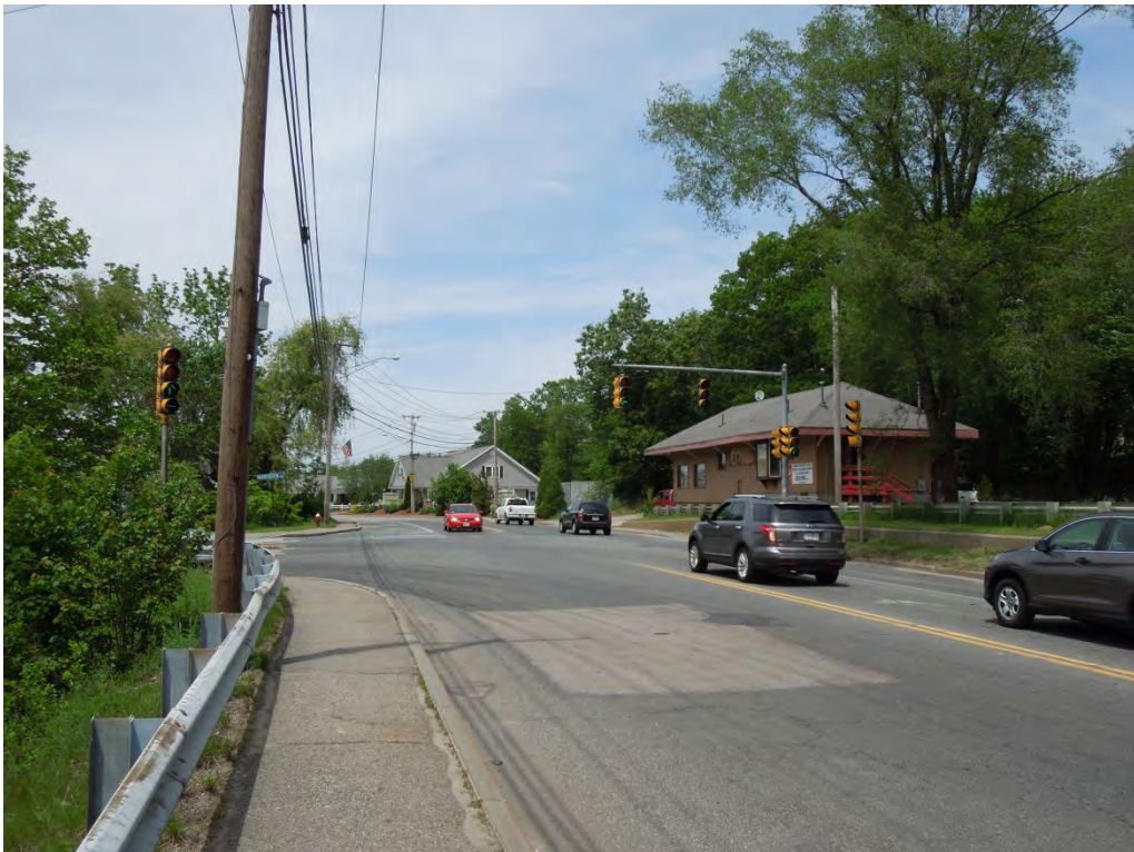
AUBURN STREET TRAFFIC SIGNAL AT BROTHERTON WAY INTERSECTION
