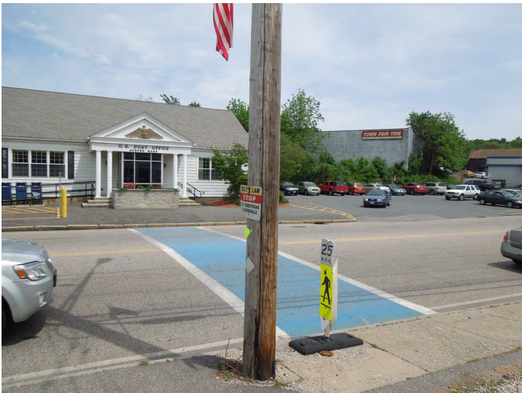
AUBURN STREET CROSSWALK AT POST OFFICE – SIGNING/ADA ACCESSIBILITY ISSUES
