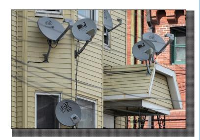
Wiring that is stapled to the siding and/ or along guttersor downspouts is also a safety concern.
