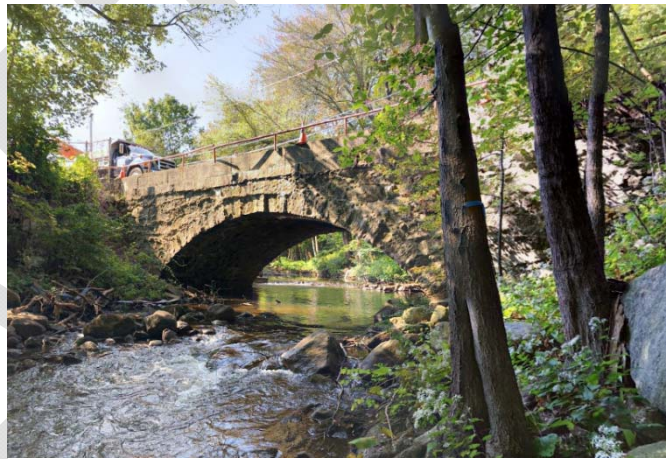
The North Street Bridge on the Mumford River. Photo: William Cundiff
