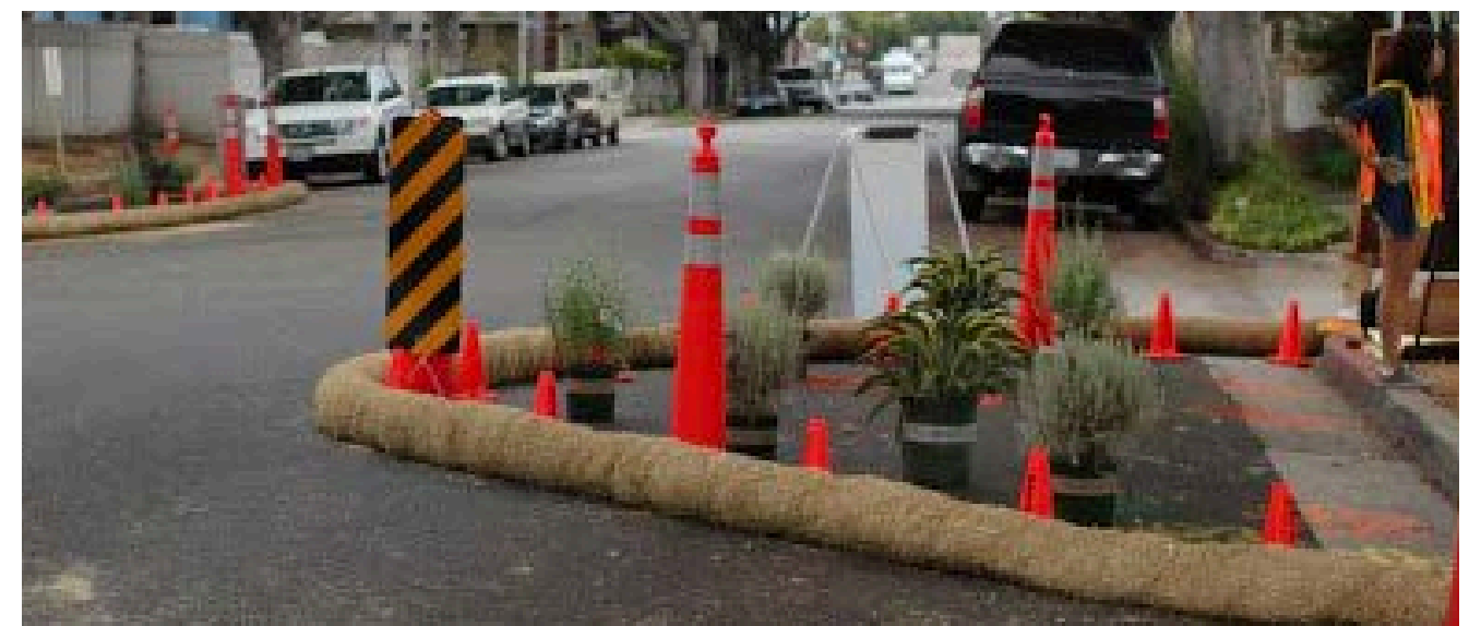
Tactical urbanism traffic calming measures using bollards, cones, and curb extensions to slow down traffic. Also, the incorporation of plants.[26]
