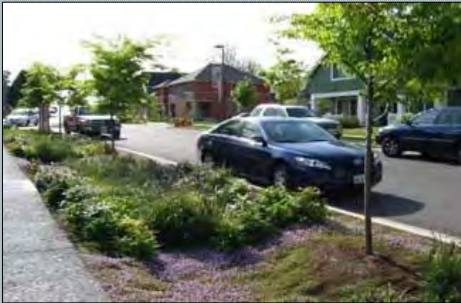
Bioswale between sidewalk and street
