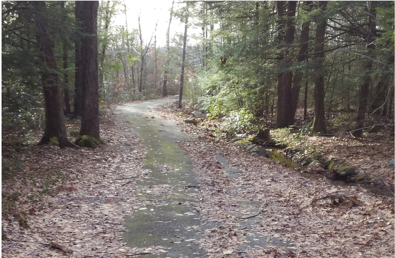
Image 8: This image shows the paved roadway down to Burncoat Pond. A proposed accessible pathway will follow this route. The Burncoat Park Sports Planning Committee hopes to remove the cracked and raised pavement, lay down an additional gravel base, and complete the path with a layer of ADA compliant stone grindings. Source: Dick O'Brien.
