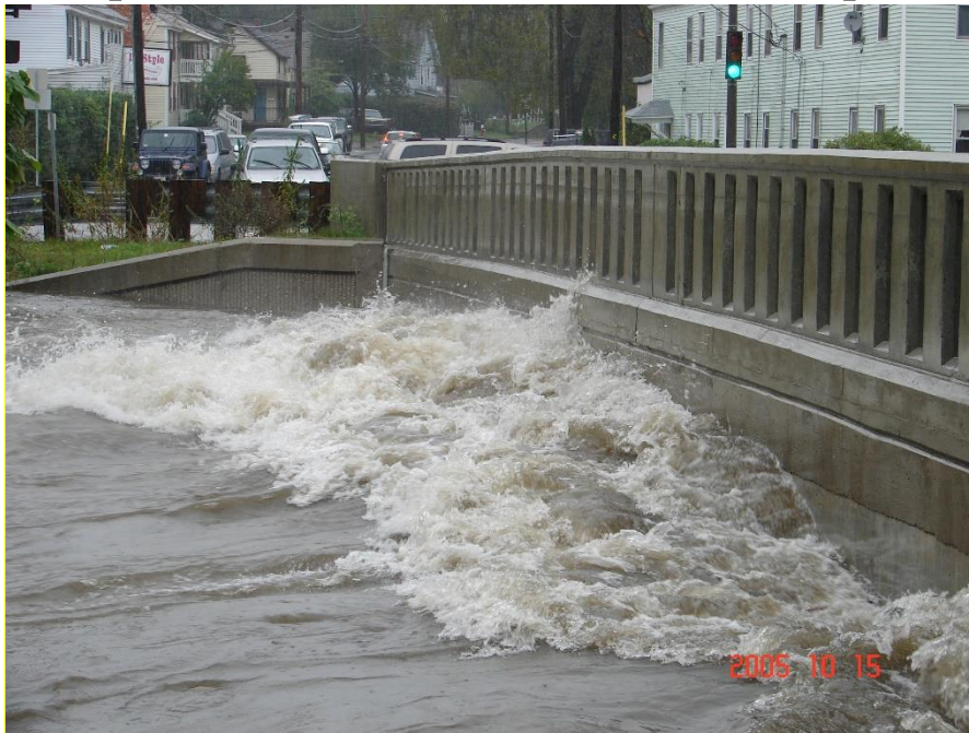
Riverlin Street, 2008 flooding, Photo courtesy of USGS
