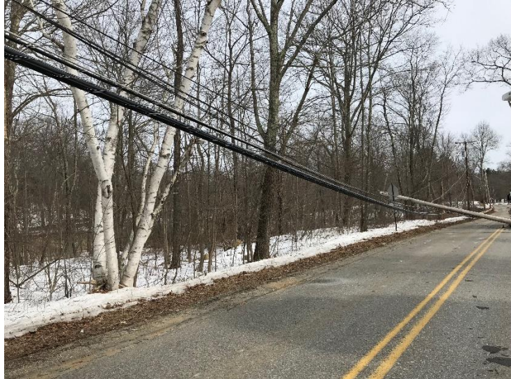
Downed power lines during 2019 wind storm
