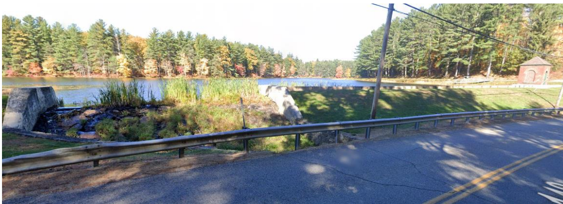
Doane Pond Dam, as seen from Google Maps Street View
