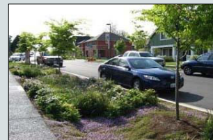
Bioswale between sidewalk and street
