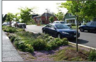
Bioswale between sidewalk and street
