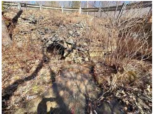
Culvert #4 – Inlet Side
