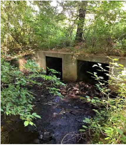
Culvert #1 – Inlet Side
