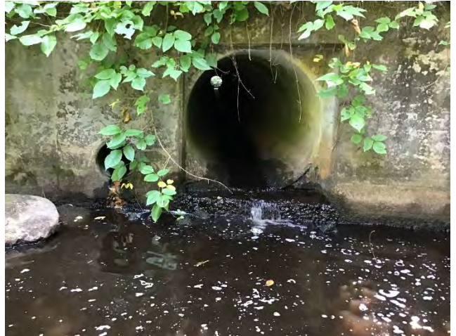
Culvert #2 – Outlet Side
