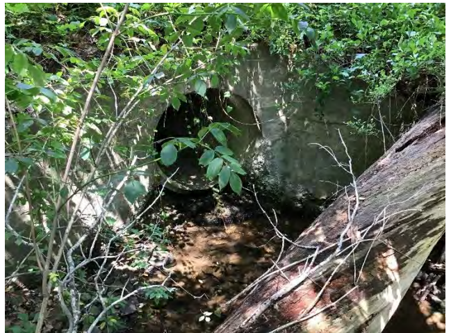
Culvert #6 – Outlet Side
