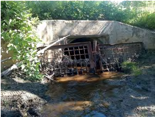
Culvert #3 –Inlet Side
