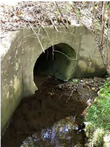
Culvert #5 – Inlet Side
