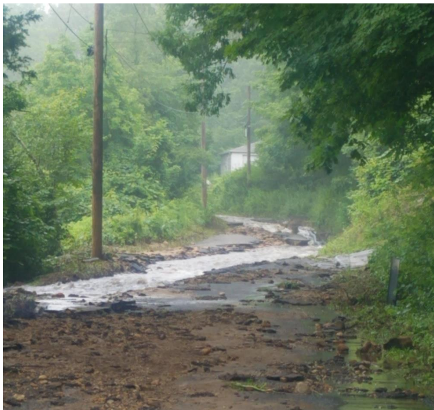
Image 4: July 2021 flooding washed out the road surface along a stretch of O'Neil Road. Photo credit: James McKeon.
