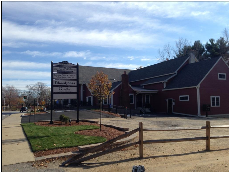
Figure 8: 419 Main Street After Redevelopment
