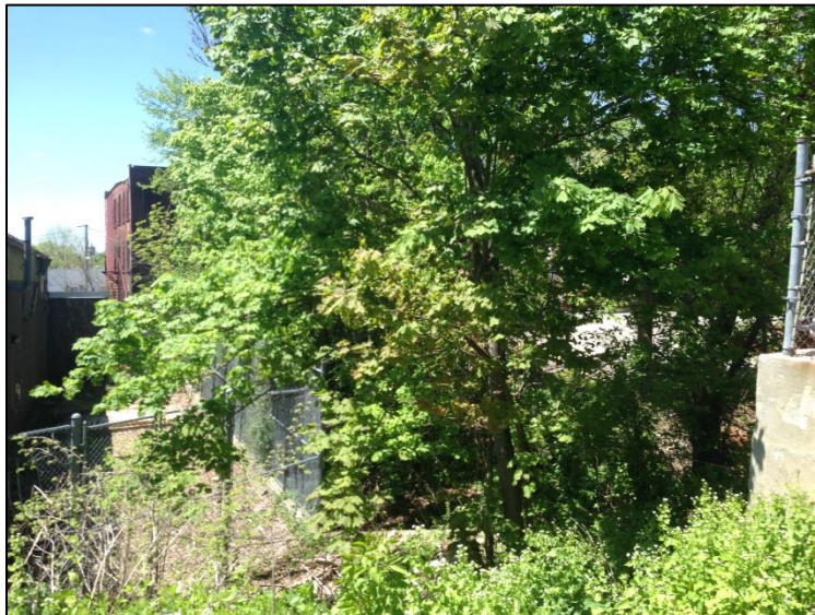
Western property line of 14 Mechanic Street
