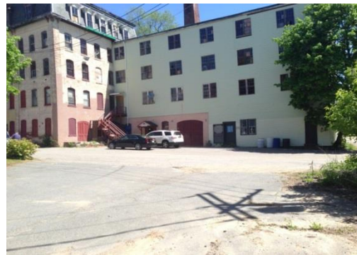
View into the rear west side of 136 Main Street
