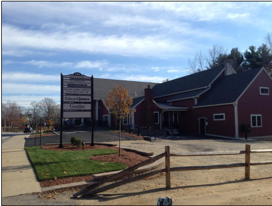
419 Main Street – mixed commercial building (formerly Basketville)
