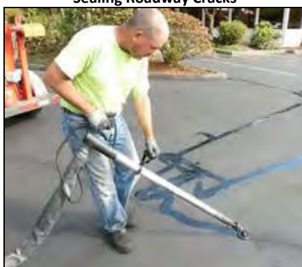
Sealing Roadway Cracks
