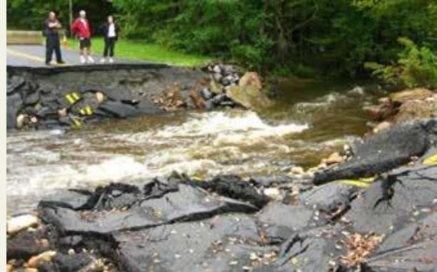
Figure 6: Undersized Crossings [2]
