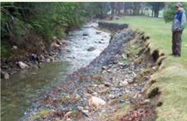
Figure 11: Scouring and Erosion [2]
