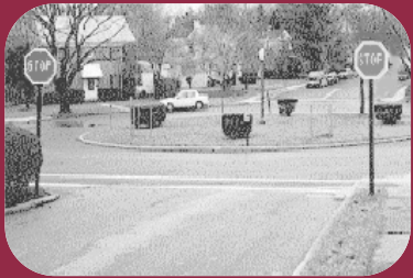
Some traffic circles use stop control, or no control, on one or more entries.
