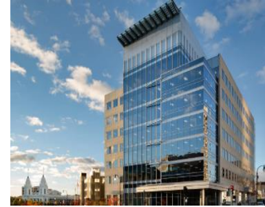
4) Commercial and Residential Buildings
