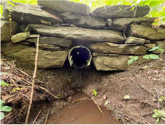
Culvert #1 – Outlet Side
