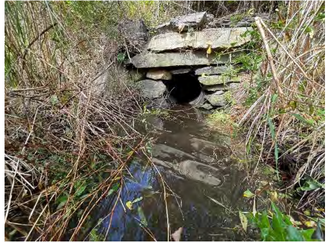
Culvert #8 – Outlet Side
