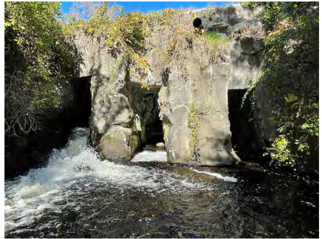
Culvert #4 – Outlet Side
