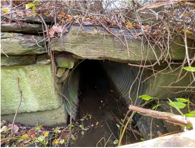
Culvert #7 – Inlet Side
