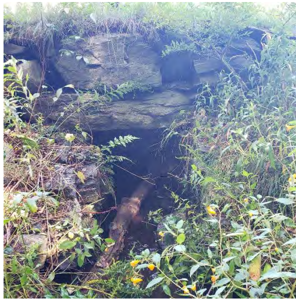
Culvert #9 – Inlet Side
