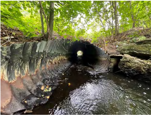
Culvert #3 – Inlet Side
