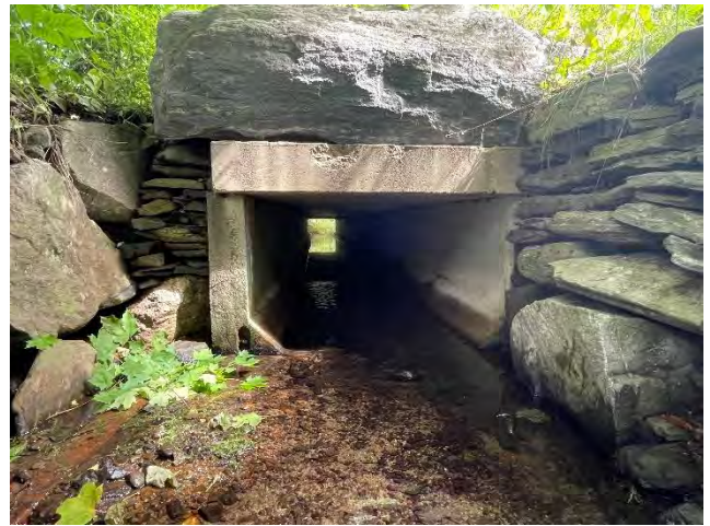
Culvert #6 – Outlet Side
