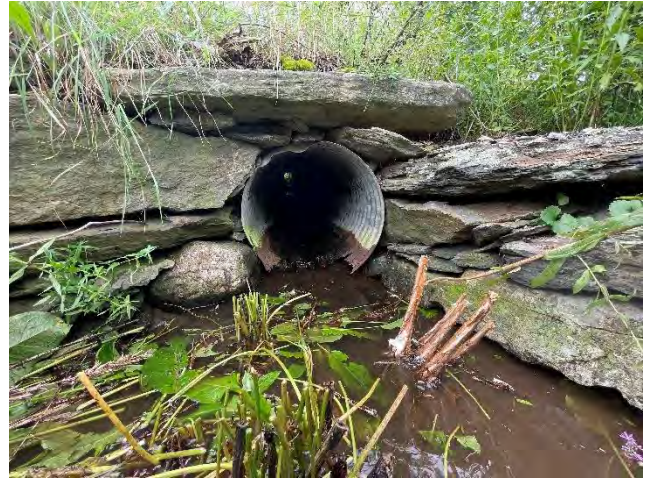
Culvert #2 – Outlet Side
