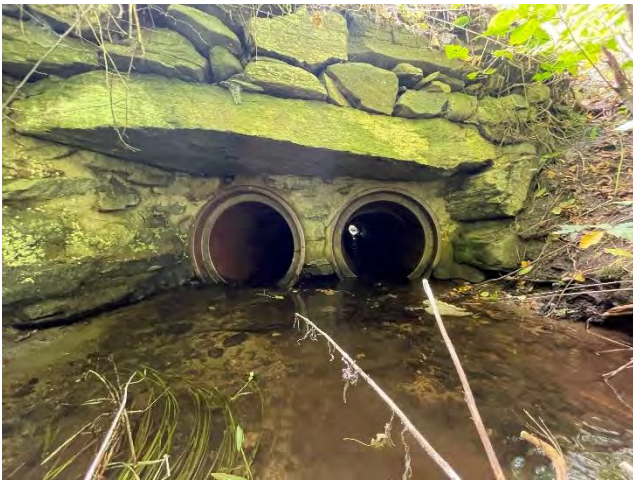
Culvert #5 – Inlet Side
