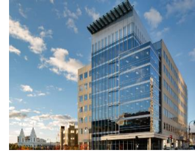
4) Commercial and Residential Buildings
