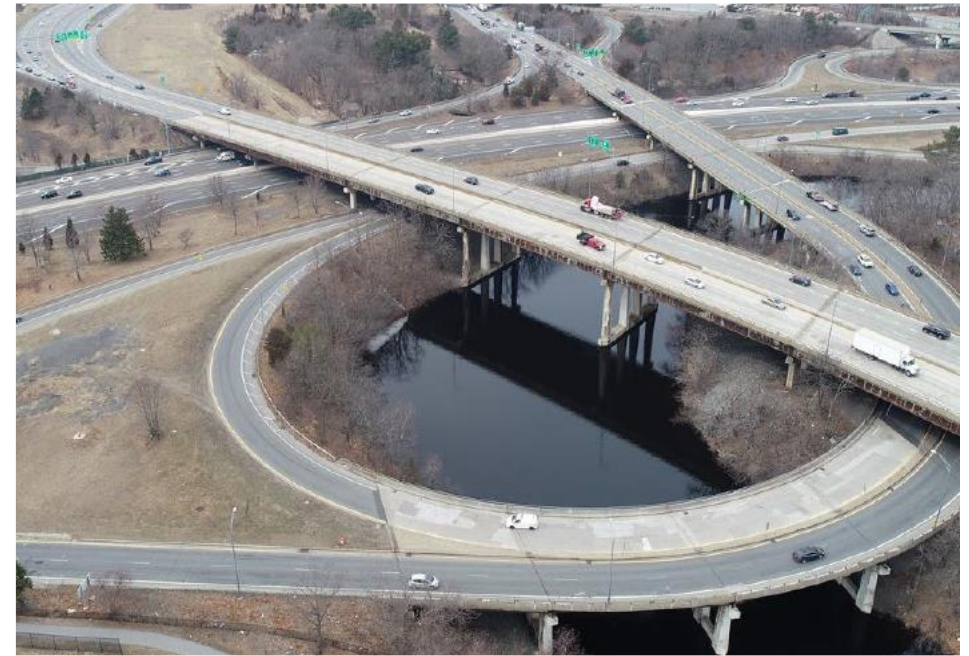
Newton and Weston – I-90/I-95 Bridge Improvements
