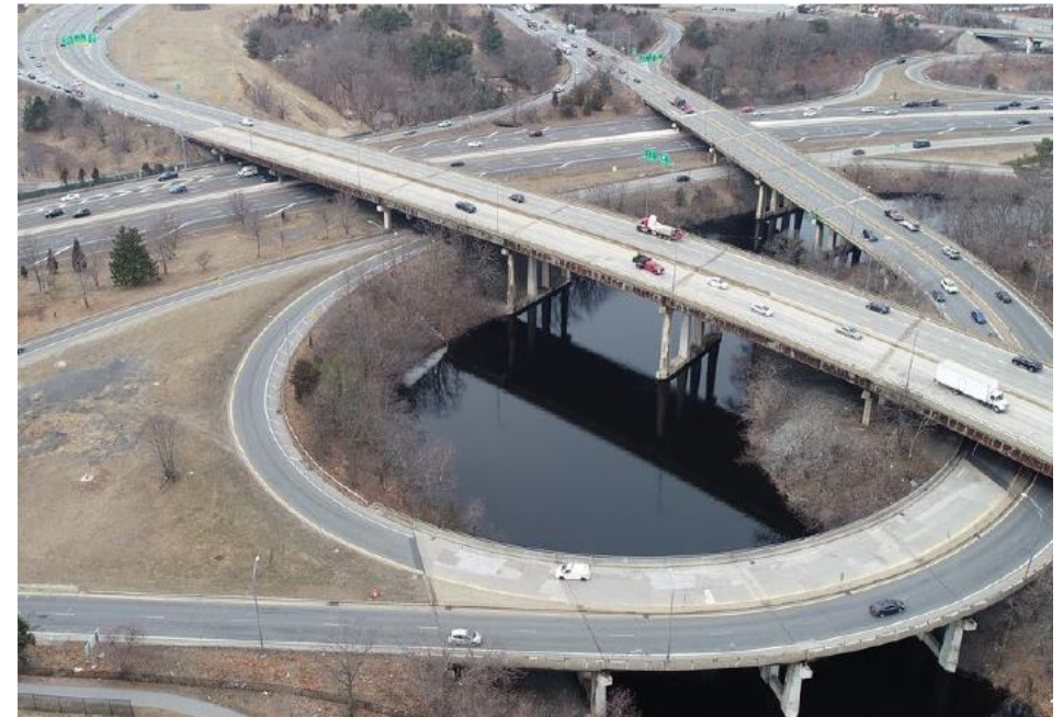
Newton and Weston – I-90/I-95 Bridge Improvements
