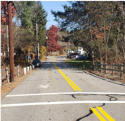
Figure 11: Crosswalk on Maple Street
