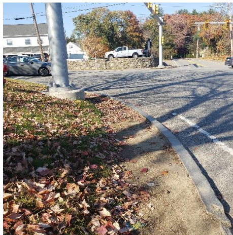
Figure 5: Tire Ruts on Bartlett Street
