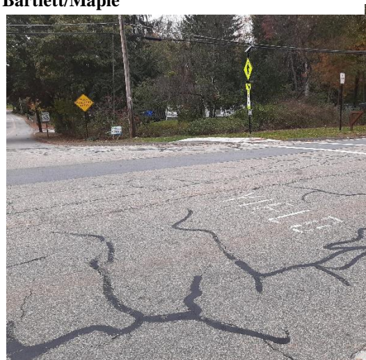
Figure 12: Truck Exclusion Sign and RRFB Crosswalk with New Curb Ramps at Bartlett/Maple
