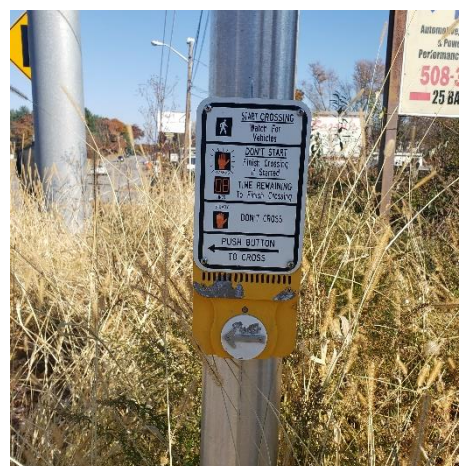
Figure 6: Controlled Pedestrian Signal
