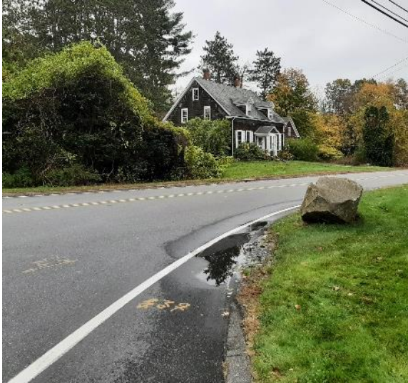
Figure 15: Potential Safety Hazard Rock Placed by Residents to Prevent Vehicles on Grass
