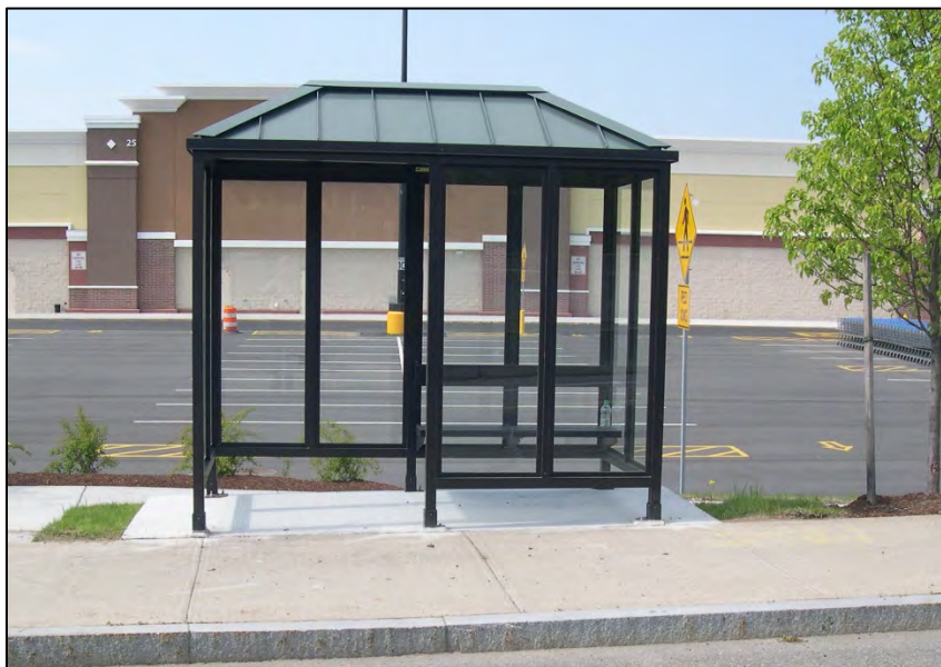
Figure IV-7: WRTA Bus Shelter
