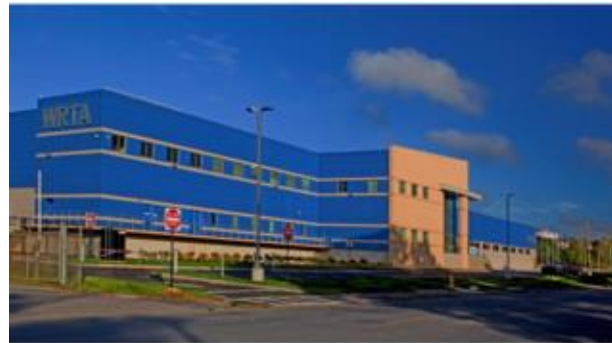
Figure IV-4: WRTA Maintenance and Operations Facility, October 2016 (source: MassTransit )
