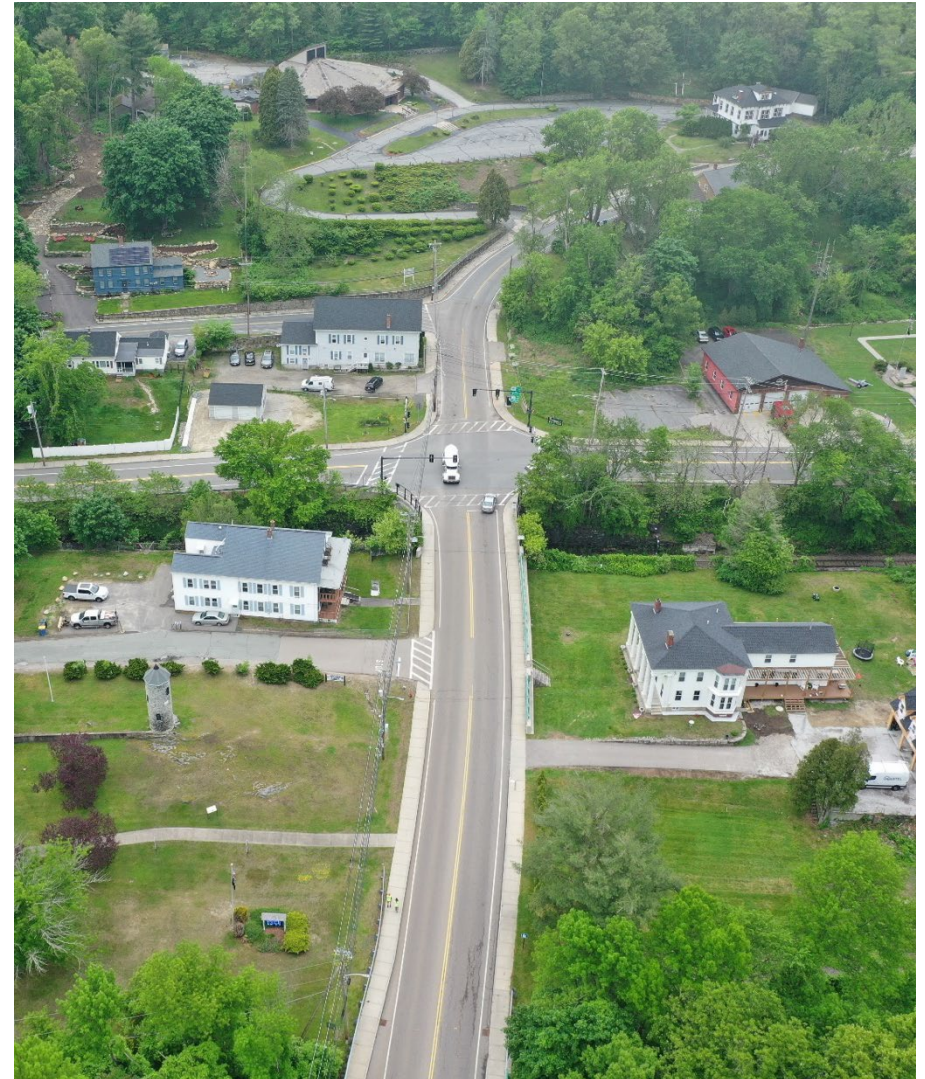
Main Street and Central Street Crossing
