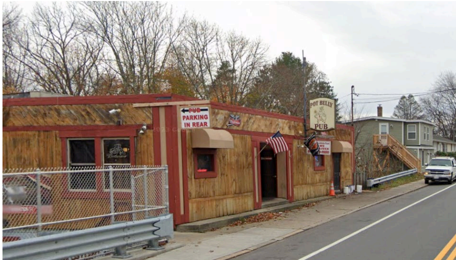
Existing non-conforming buildings in the village center with little-to-no setbacks.
