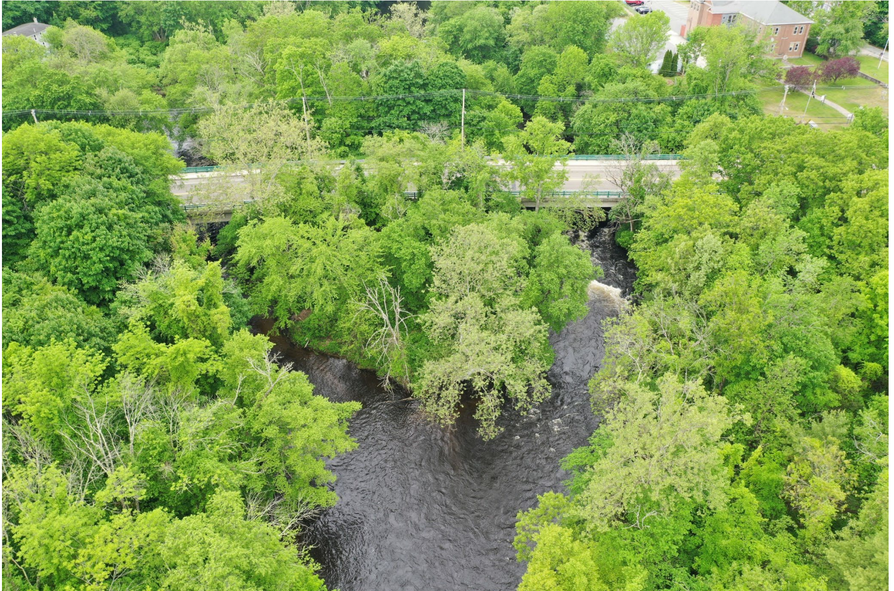
Central Street Bridge Crossing the Blackstone River
