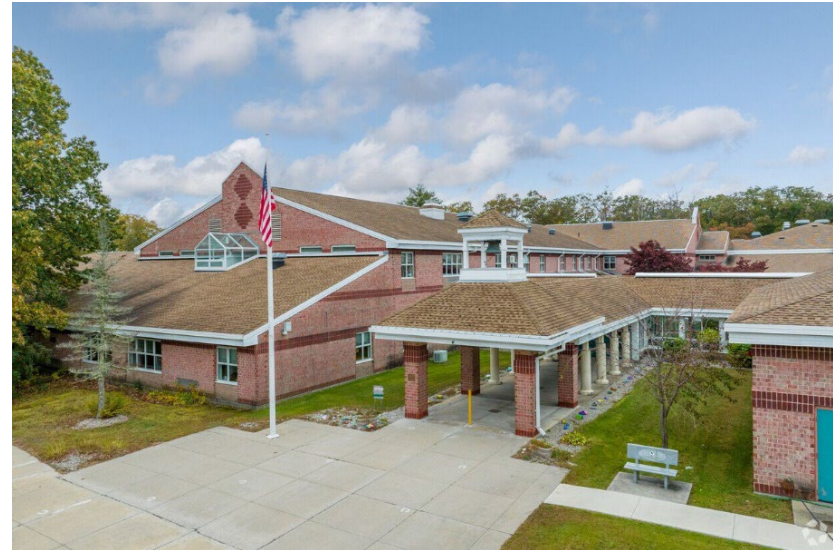
Millville Elementary School
