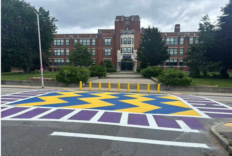
Painted intersection - Increases visibility
