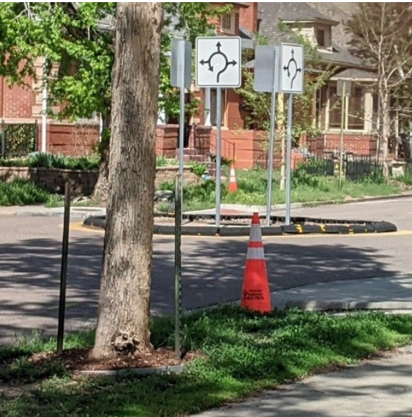
Neighborhood traffic circle – Reduces speeds and traffic conflicts
