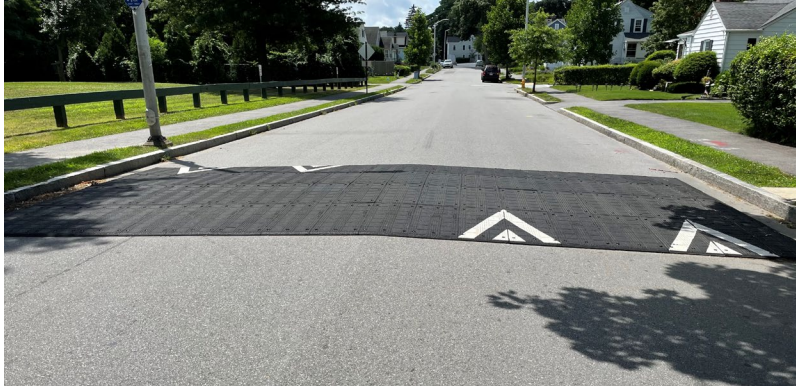
Speed Hump – Reduces speeds
