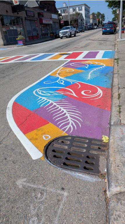
Painted curb extension and crosswalks – Increases visibility
