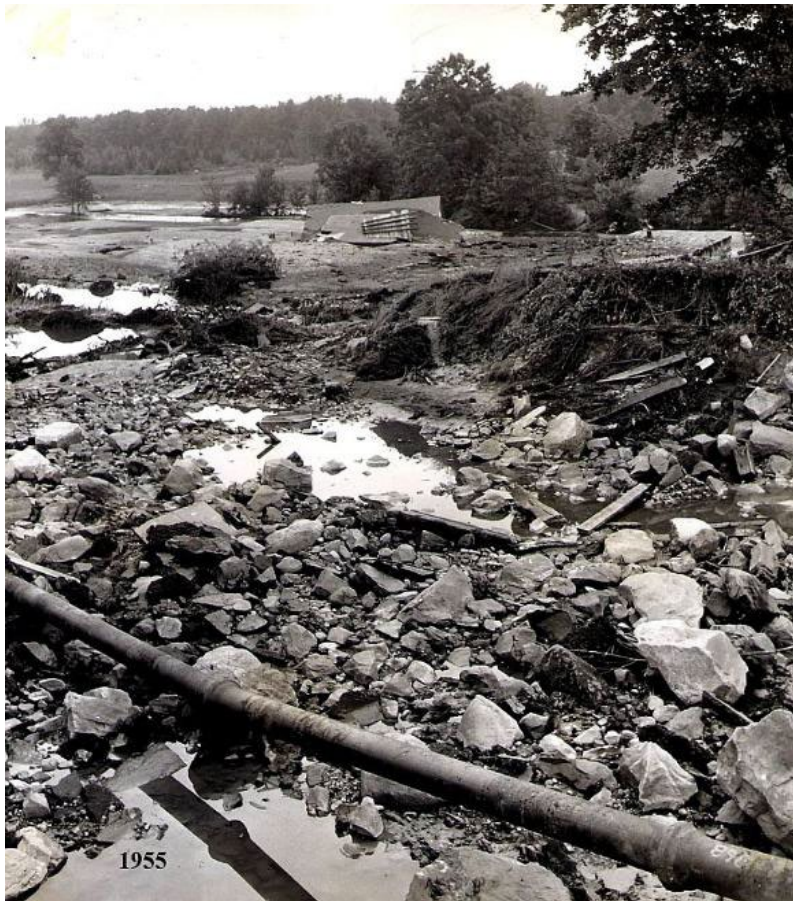
Images 1 and 2: Photos of the aftermath of the major flooding event in 1955 which occurred in Blackstone after Tropical Storm Connie and Tropical Storm Diane hit the Town in succession
